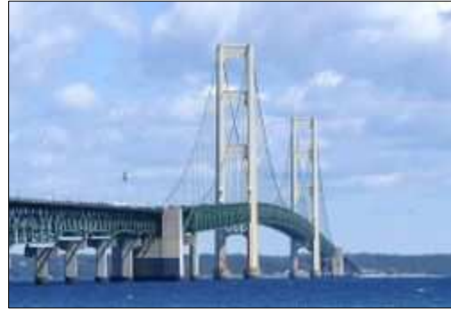
Northern Michigan's Mackinac Bridge
